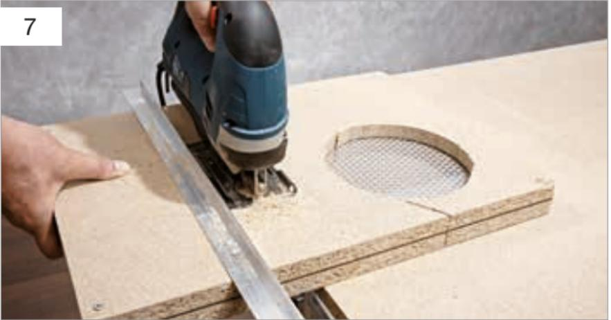
For straight cuts, you can screw on an aluminium bracket as an end stop for a super-straight cut.
