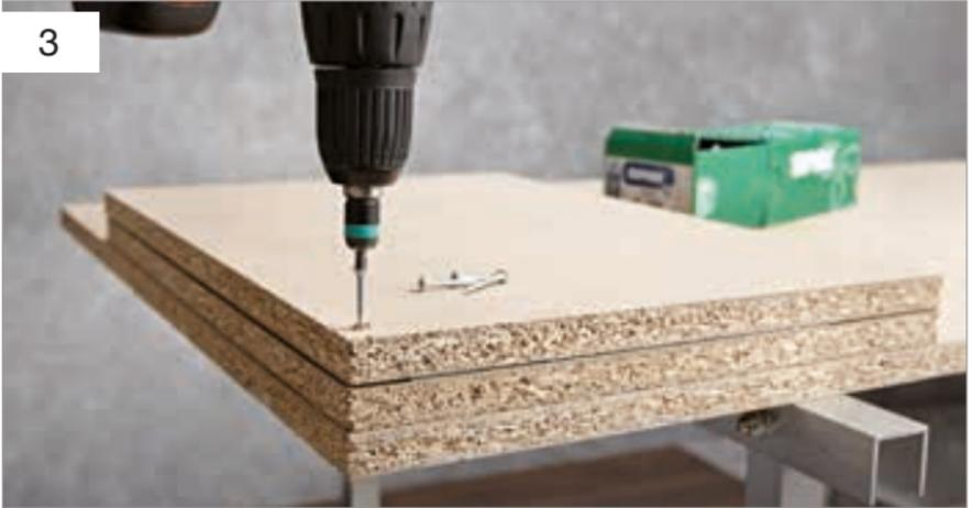
Now use countersunk screws to connect the two wooden boards. You can also drill through the part of the sheet that is not required and fix it with screws so that it cannot slip out of place.
